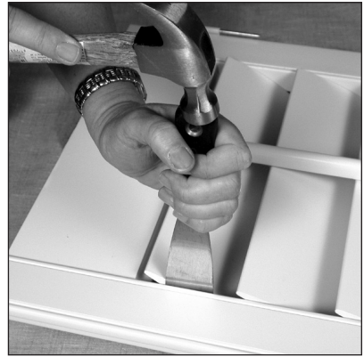
Replacement Louver Pin Spring-loaded for louver replacement
